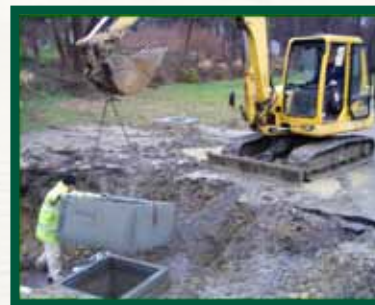
Ledgebrook Ln. Installed 120' storm sewer pipe & 3x3 catch basin.
