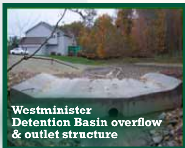
Westminister Detention Basin rebuilt outlet
